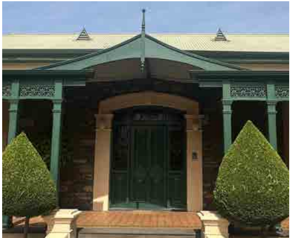
Figure 10: 1980s reproduction verandah detailing on 99 Palmer Place
