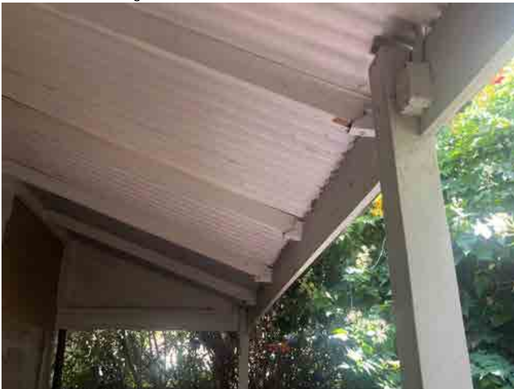
123 Barnard Street non-original verandah
