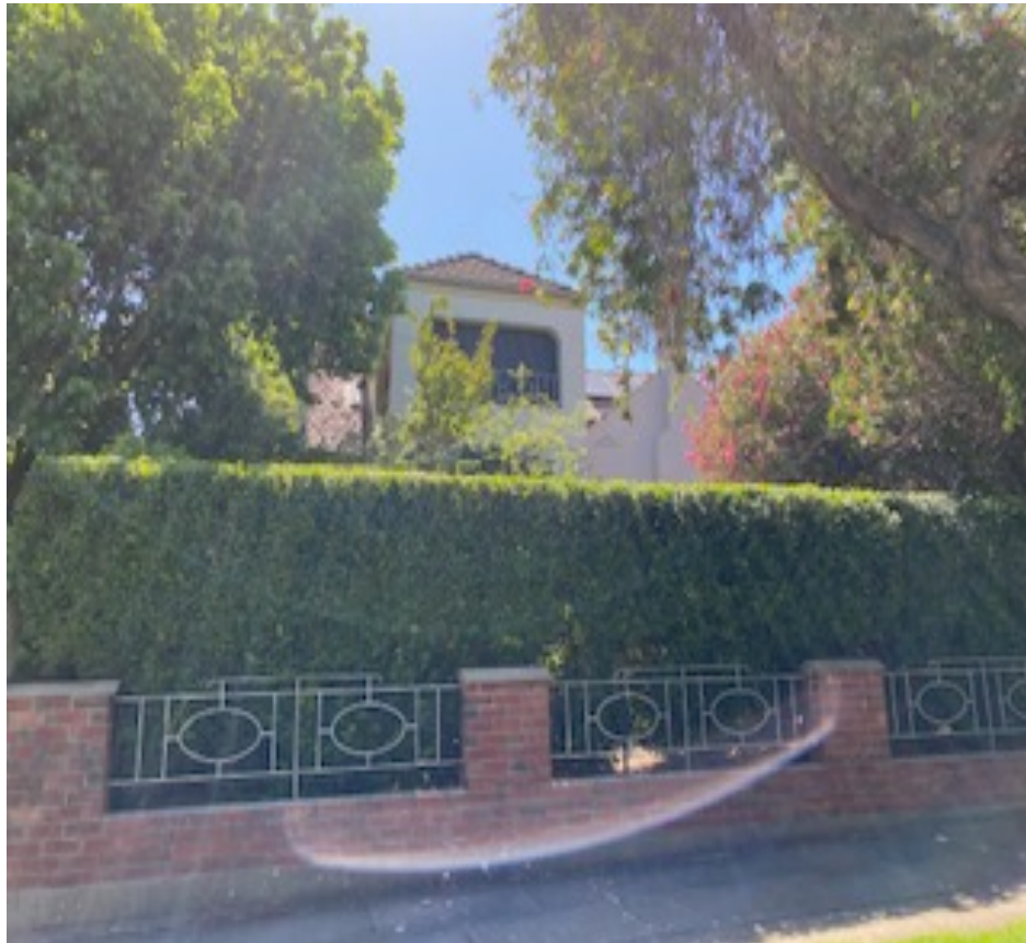
66, Mills Terrace: The Subject Property
